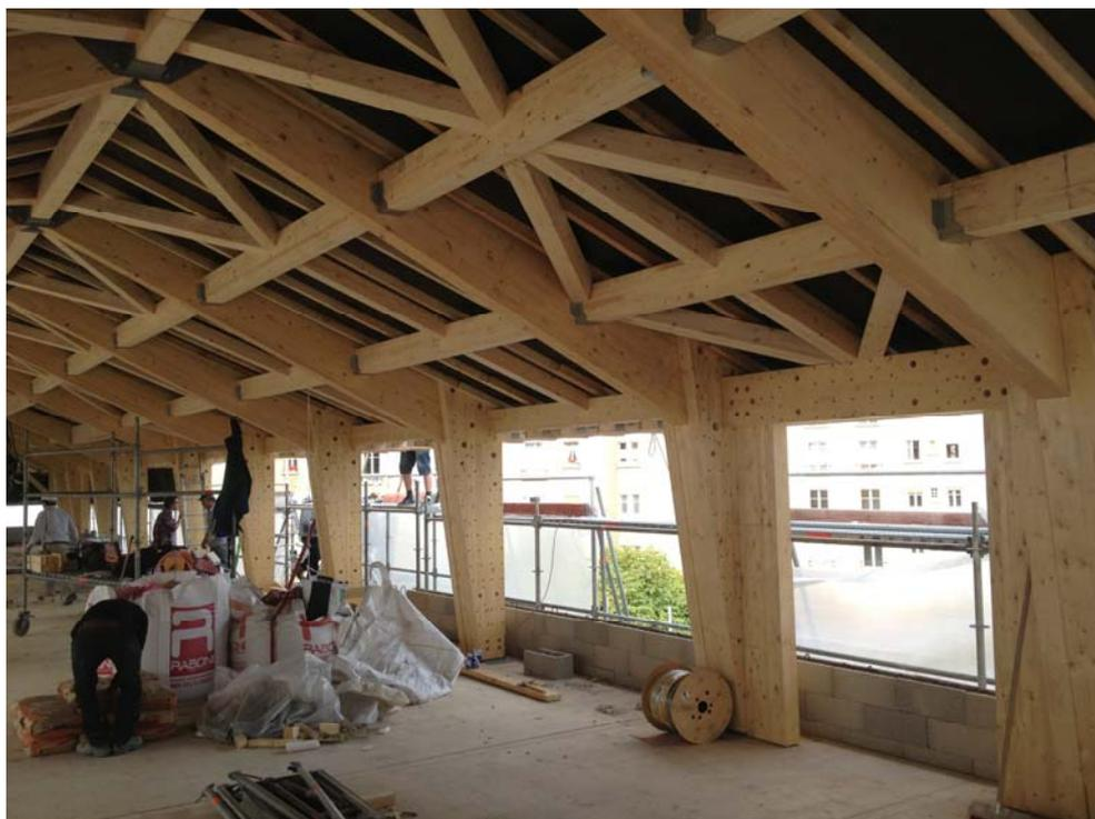
Image 18: Fin de pose de la charpente / © Barcque Charpentes
