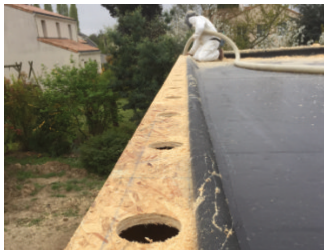
Insufflation fibre de bois
